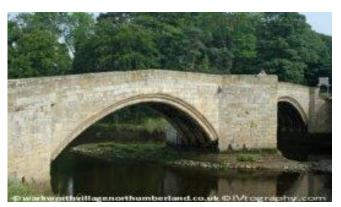
There are two bridges over the River Coquet at the north end of the village at Warkworth. The first is the old medieval bridge which was built in the last quarter of the 14th century (it is suggested that the actual date of construction was 1379). It has two 60 feet (18.28m) span segmental stone arches each with double arch-rings, and four ribs.
