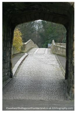
The bridge is one of only two fortified medieval bridges in Britain (the other is in Monmouth) and it is a Scheduled Monument and a Grade II Listed Building. In 1859 the bridge was described as being founded on both rock and wooden platforms with the north abutment being built on stone and the south on a timber platform.
